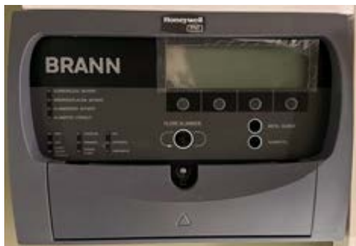
Figur 2 Brannmanspanel
